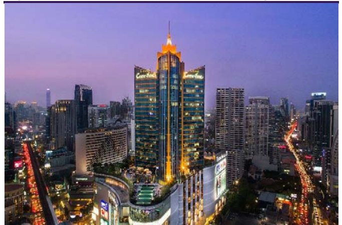
Figure 2: GCPT21 is adjacent to shopping malls
